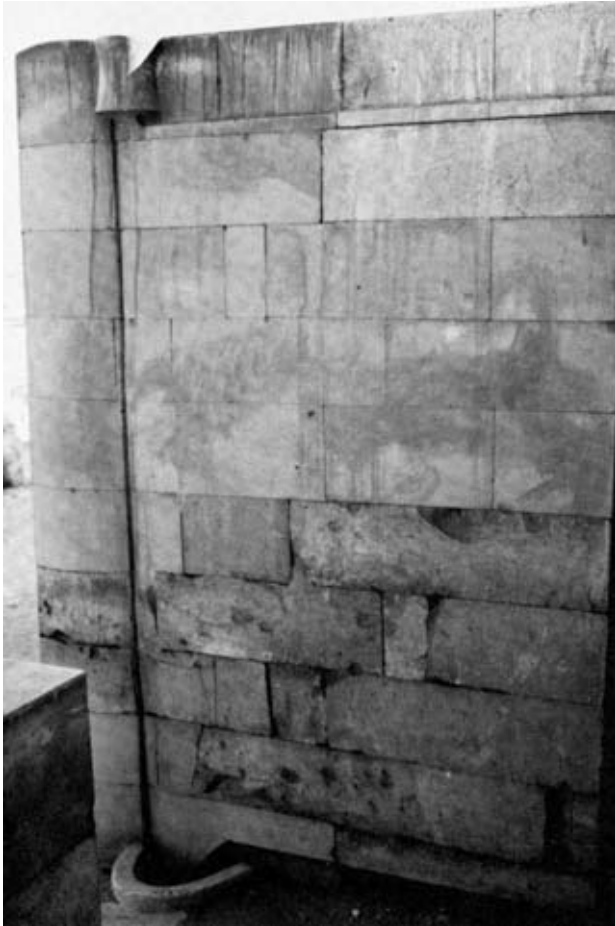
Fig. 6 Opened door with hinges and sockets modeled into a limestone structure in the Heb-Sed court of Zoser at Saqqara, Egypt, circa 2750 B.C.
