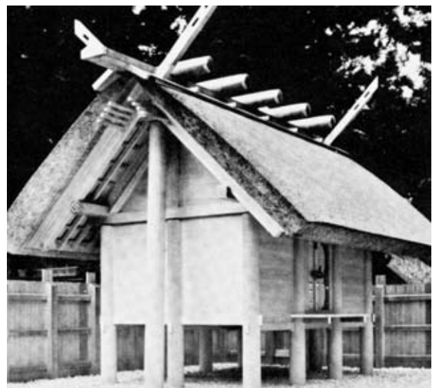
Fig. 15 Ise Shrine, West Treasure House with five katsugi on the roof peak. Photograph by Yoshio Watanabe.
