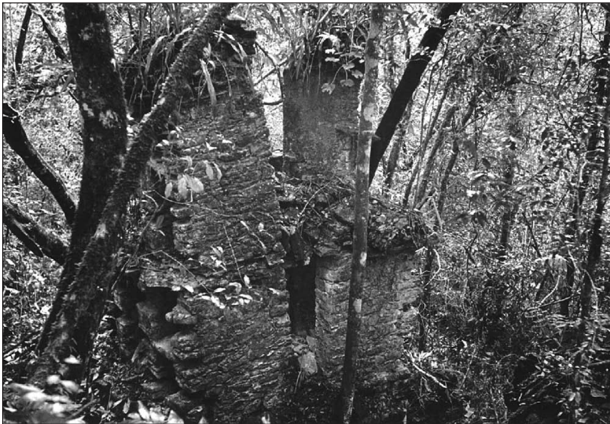
View of roof comb on Structure 6
