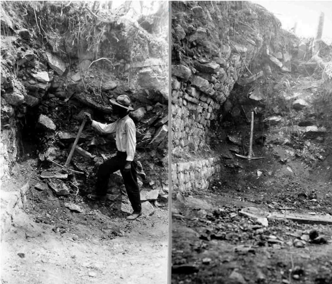
Figure 9.9. Clearing the outer chamber of Structure 1B-3: Left—start of excavations; right—halfway through clearing. Note the remaining section of the corbelled vault
