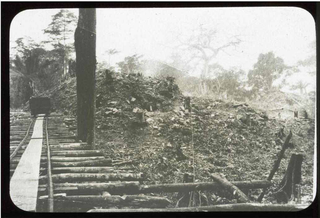
Figure 1.17. The narrow-gauge rail track constructed to remove debris from Quirigua Structure 1B-1 in 1912. The mound shown is 1B-1 before excavation.
