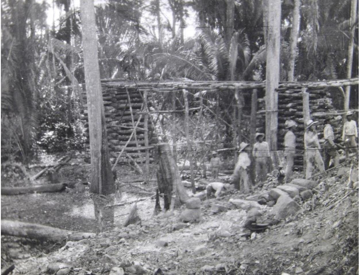
Figure A.15. Before actual excavations could begin, the SAA team had to construct a trestle upon which to lay a narrow-gauge rail track for the purpose of carrying excavation debris away to a dump site. The height of the trestle shows the elevation of Structure 1B-1 above the plaza floor.
