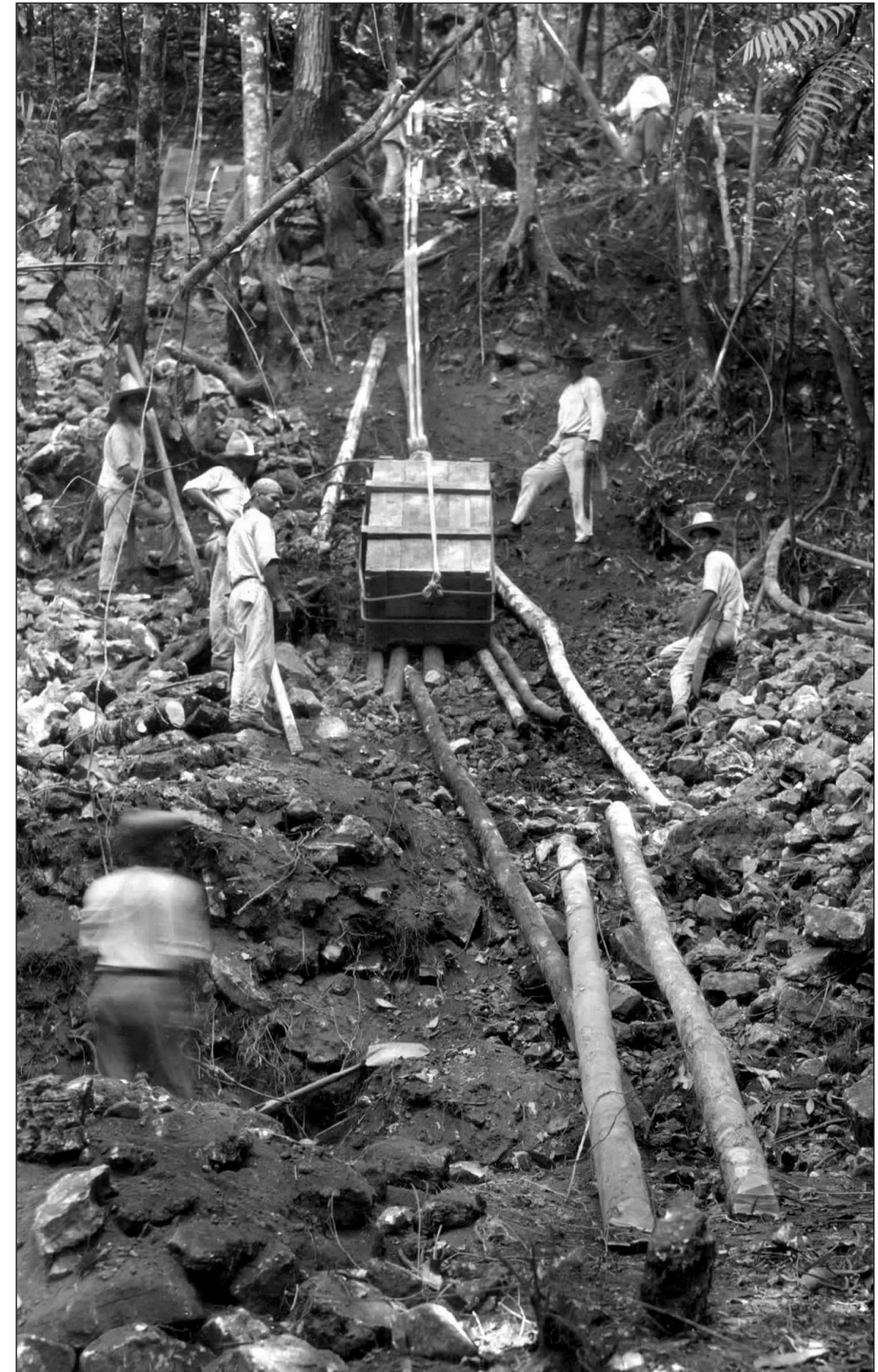
Pulleys are used to drag a monument boxed in a mahogany crate uphill (Piedras Negras Archives 31-161).
