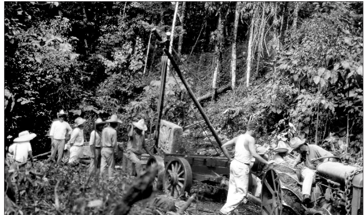
Removing monument with makeshift pulley and tractor (Piedras Negras Archives unnumbered).
